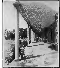
SOUTH PORCH OF NEW FIREPROOF BUILDING
